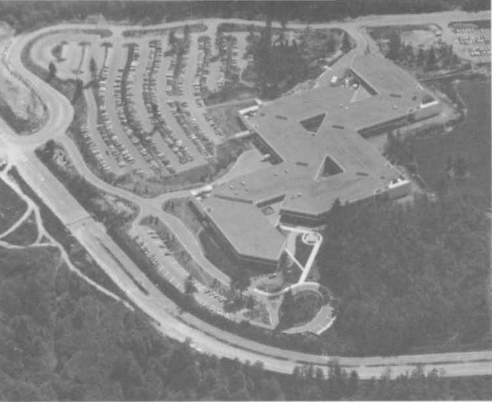
Fluke Corporate Headquarters, Everett, WA, U.S.A.
